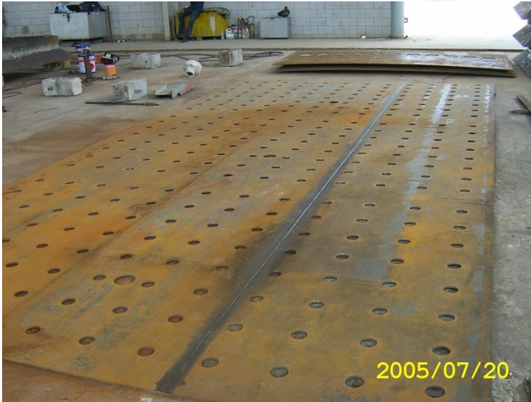
← Long Butt Joint Welding
